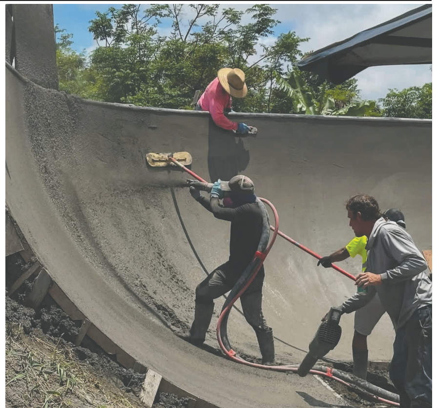
Volunteers work under time pressure to smooth the concrete perfectly before it sets up.
